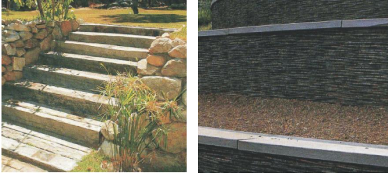
USE OF TIMBER STEPS AND INNOVATIVE TIMBER RETAINING STRUCTURES.
